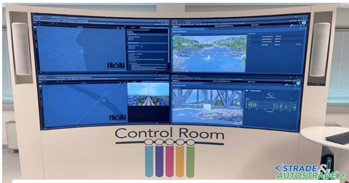
3. Demo Center Almaviva: la Control Room MOOVA
